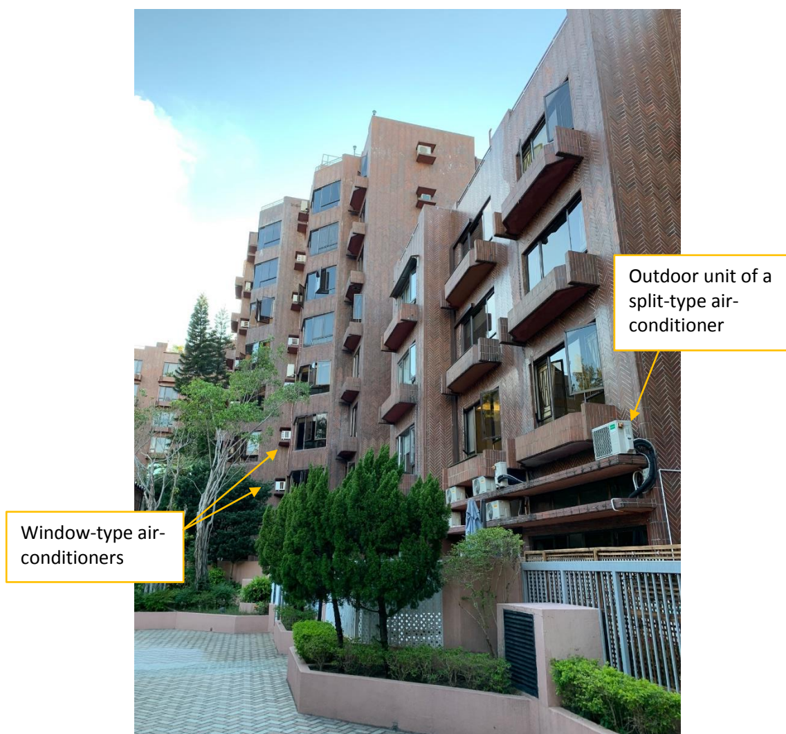
Figure 1.4 A residential development where a mix of split and window-type air-conditioners are in use
