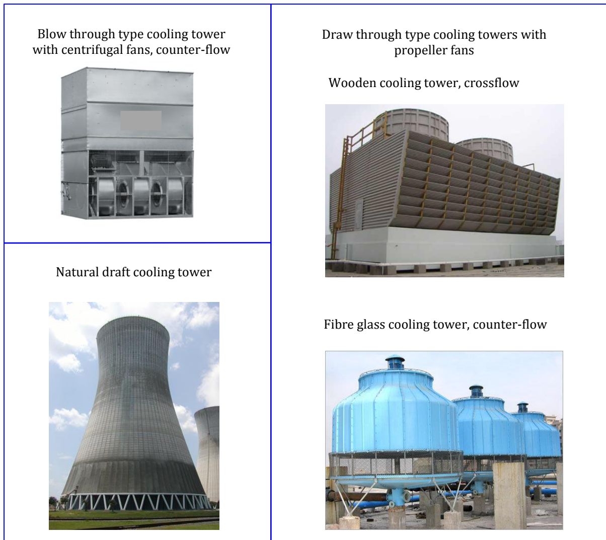
Figure 6.15 Types of cooling towers
