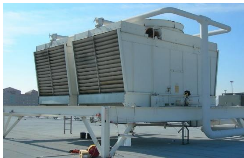
c) Cross-flow cooling towers
