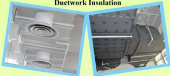
Duct Support Insulation (DSI)
