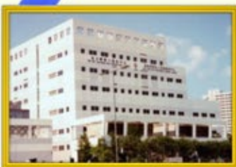
General Cancer Centre, Prince of Wales Hospital Shatin, N.T. Year of Completion : 1994
