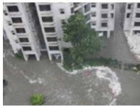
Underground car park was completely flooded
