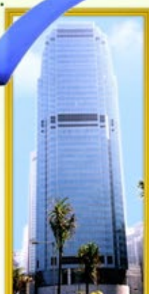
International Financial Centre Phase I (IFC-I) South West Tower at Hong Kong Station, H.K. Year of Completion : 1998
