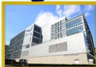
Central Mail Centre Kowloon Bay, KLN. Year of Completion : 2013
