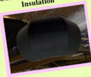
Pipe Support Insulation (PSI)
