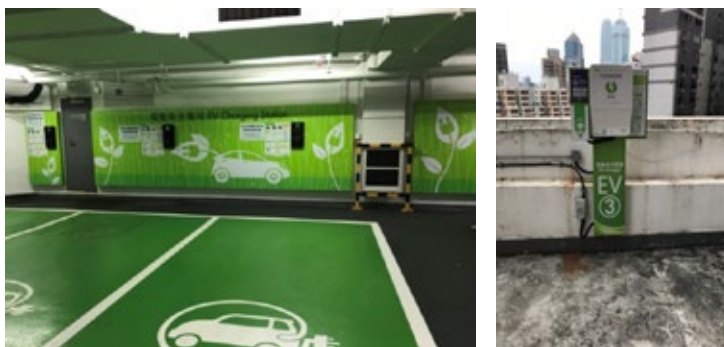
EV chargers installed in commercial and residential buildings
