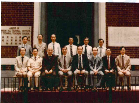
Hong Kong Technical College before the demolition in June 1986 with Dr. Ching Yuen-Kai (Retired Principal)
