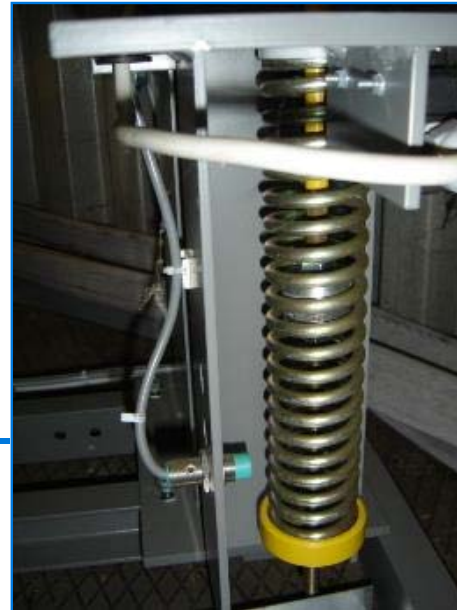
Rope brake actuated (tripped by CPD)
